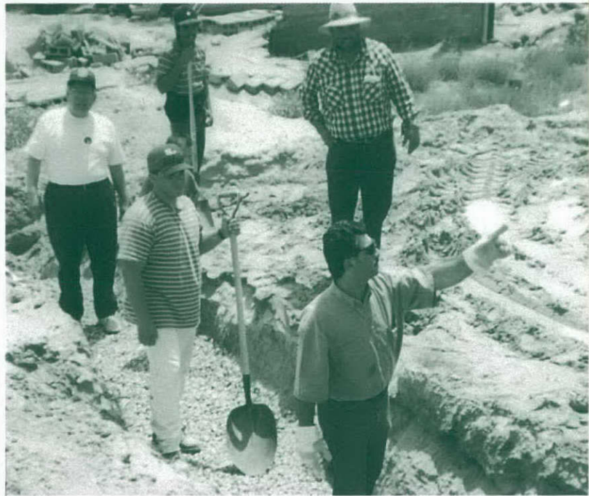
Colonia families work to build septic system.
