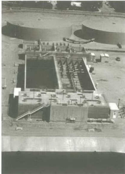
Brawley's treatment plant near completion.
