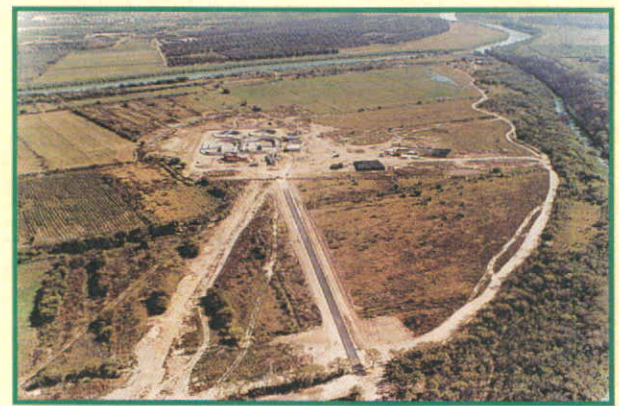
Construction of Wastewater Treatment Plant of Piedras Negras, Coahuila
