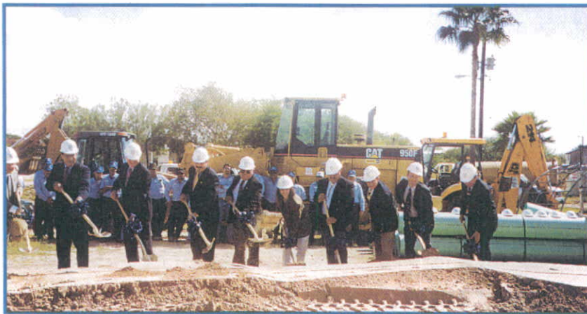
The ground-breaking ceremony for the wastewater project of Roma, Texas in October, 1999
