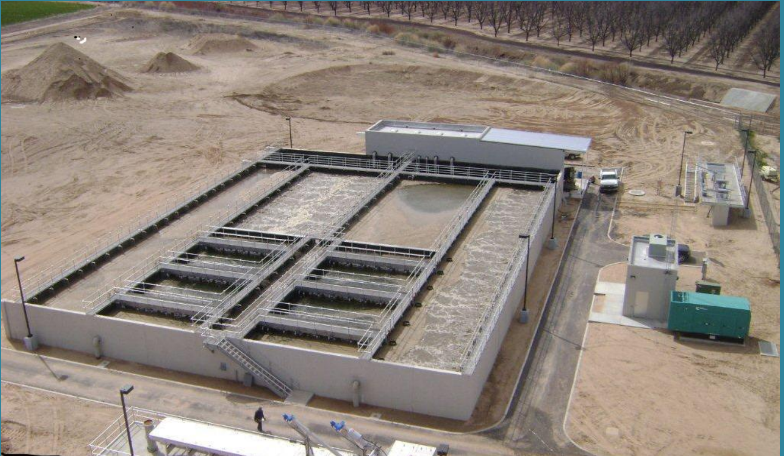
Wastewater Treatment Plant in Fabens, TX. with 1.2MGD capacity
